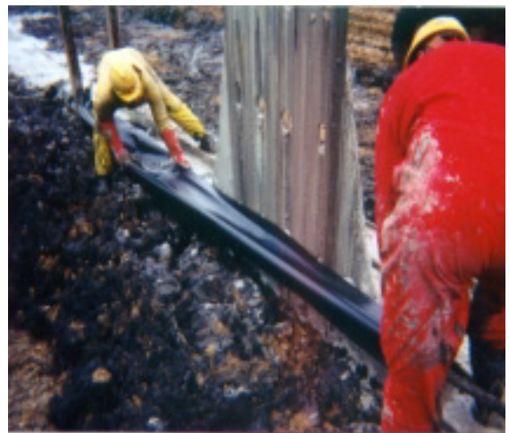
Figure 9. Geomembrane Wall Installation
