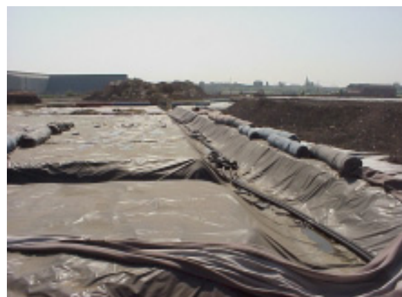
Figure 6. Geomembrane Cap Construction
