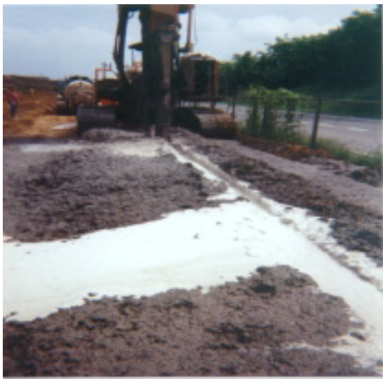
Figure 7. Bentonite-Cement Wall Installation
