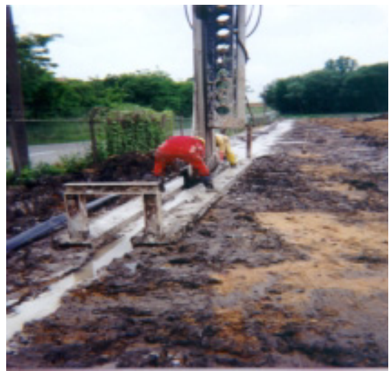
Figure 10. Geomembrane Wall Installation
