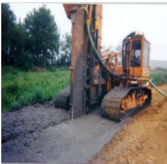
Figure 8. Bentonite-Cement Wall Installation
