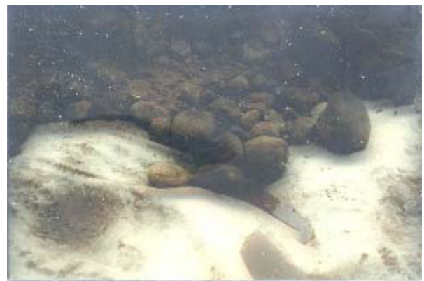
Figure 7. Geotextile stressed by deformation caused by granular fill material on soft subsoil (Wetting 2002).
