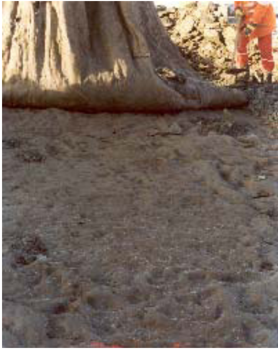
Figure 22. Extraction of geotextile SNP 4E.
