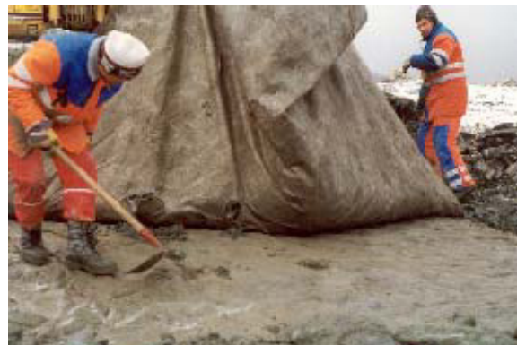
Figure 21. Extraction of geotextile, CTP 4D.
