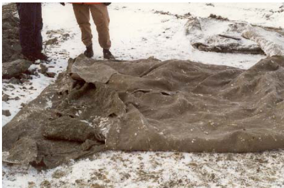
Figure 9. Geotextile with severe damage from tearing (SINTEF report 1997).
