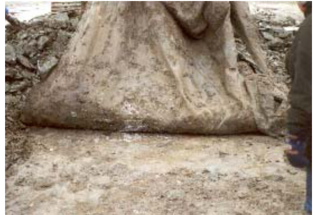
Figure 20. Extraction of geotextile CNP 4A.
