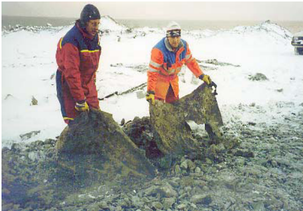
Figure 23. Extraction of class 2 geotextiles.
