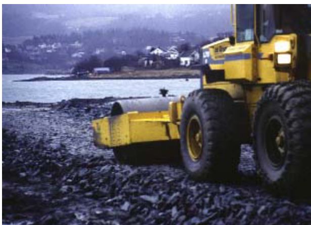
Figure 19. Compaction of fill.
