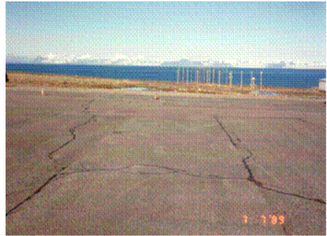
Figure 7 Reflective cracking of asphalt overlay on concrete pavement, Svalbard, Norway
