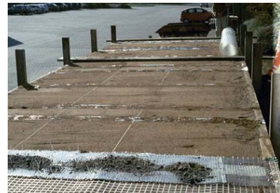
Figure 17 Installation of geogrid in test bin
