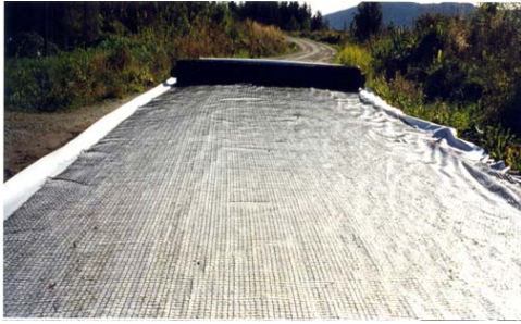
Figure 14 Hitra, Norway. Installation of geogrid
