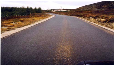
Figure 15 Hitra, Norway, Road after installation of asphalt overlay
