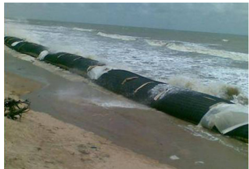
Figure 5. Geotextile tube at Shankarpur, West Bengal, India.
