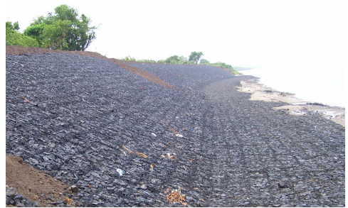
Figure 7. Revetment by Polymer rope gabions in Narmadha river at Madhi, Gujarat.
