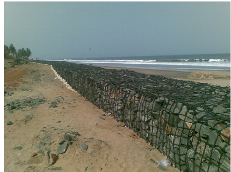
Figure 4. Geotextile tube covered with armour layer of polymer rope gabion.
