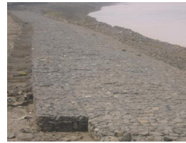
Steel Gabion as revetment
