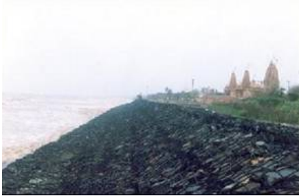
Figure 2b. Sea wall with polymer rope gabion protecting sea-shore (Tithal, Gujarat)
