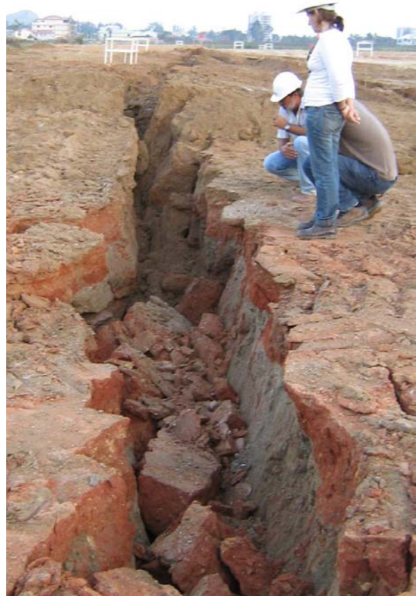
Figure 6. Embankment failure: (a) location showing the haul road (b) fissure developed at the embankment.
