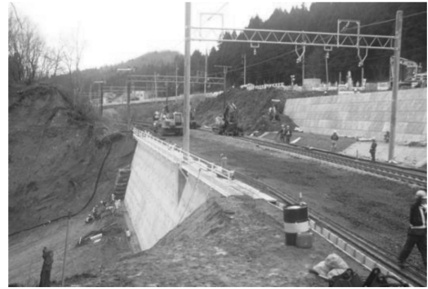
Figure 4. Reconstructed GRS-RW with full height rigid facing.
