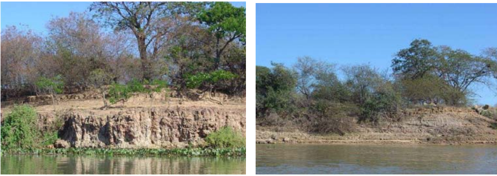
Figures 5 and 6. Erosion in the margins of San Francisco River
