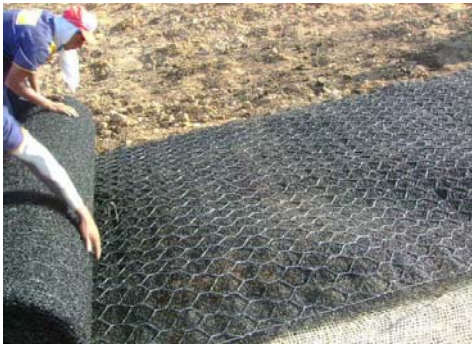
Figure 11. Geomat being unrolled on the slope Figure 12. Geocomposite protection installed on the slope
