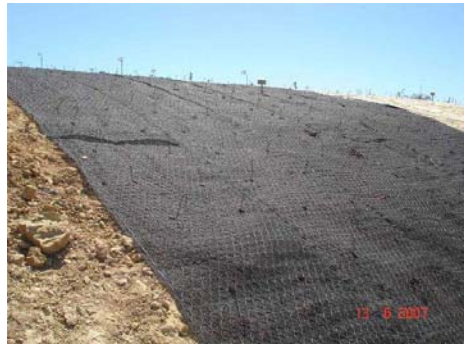
Figure 11. Geomat being unrolled on the slope Figure 12. Geocomposite protection installed on the slope
