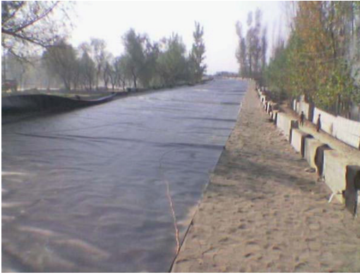
Photo 5. Photograph showing installation of geomembrane.
