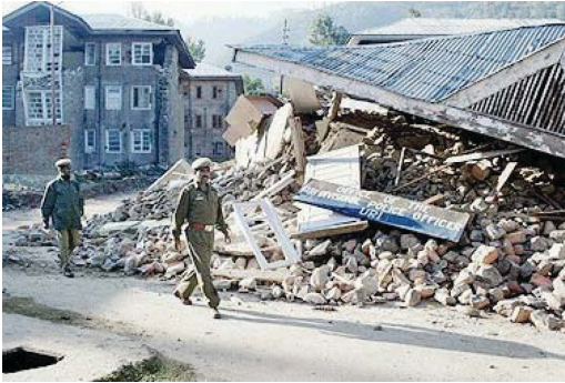
Photo 2. Damaged building at Uri about 30 km from the construction site.
