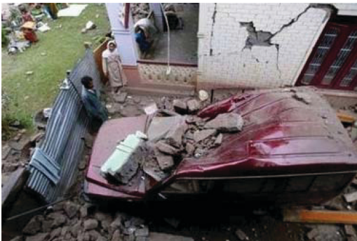
Photo 3. Damaged building near the construction site.
