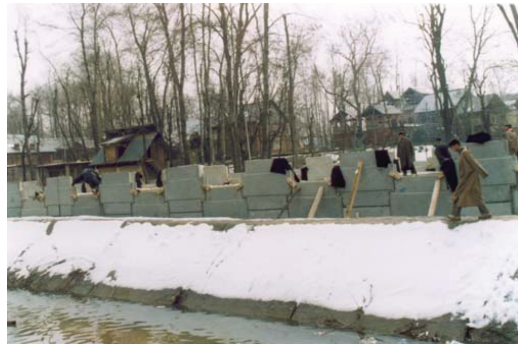
Photo 4. Reinforced soil wall running parallel to the canal.
