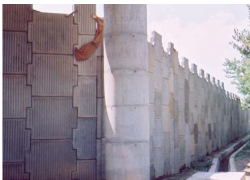
Photo 1. Reinforced earth wall for bridge no. 127.
