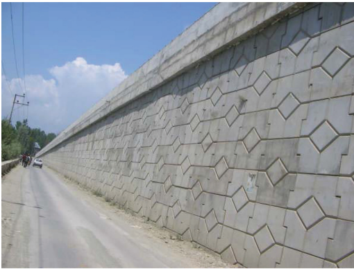
Photo 6. Photograph of completed structure of Bridge No. 165.
