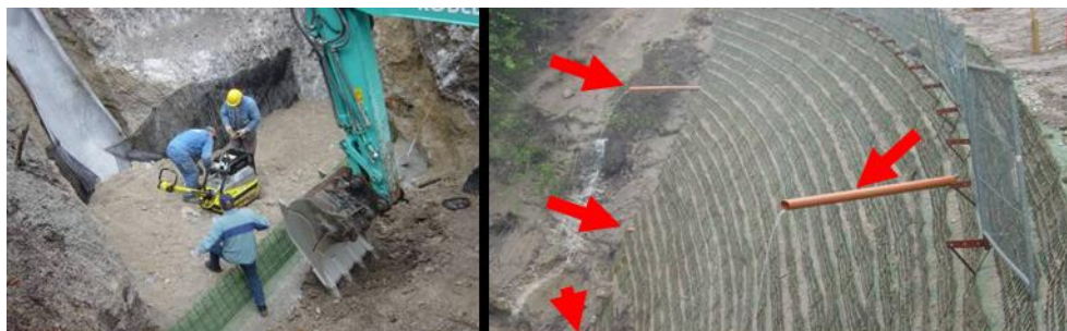
Figure 5. Foundation and drainage works
