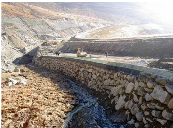
Figure 9. Site view of the protection bund Diasbachalpe
