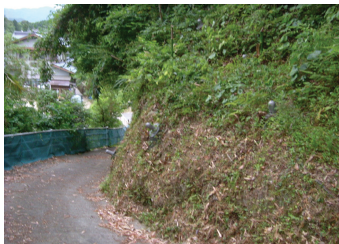
Photo 1. Treated slope by Non-frame method in Fukuoka.
