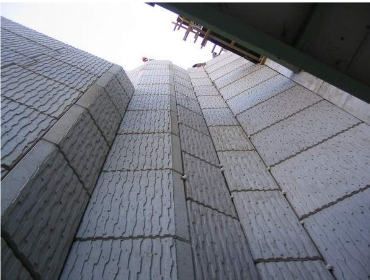
Figure 7. The highest section H=22.5\text{m} of the “PRS” wall next to the crusher
