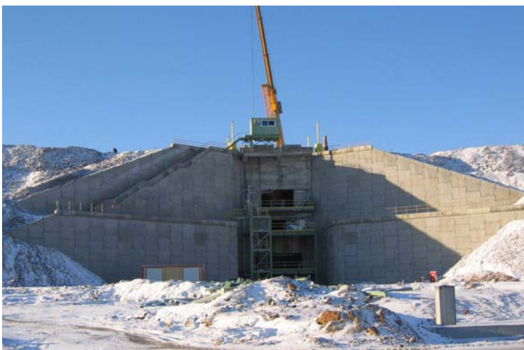
Figure 1. Wing walls of the crusher wall, H=22.5m.
