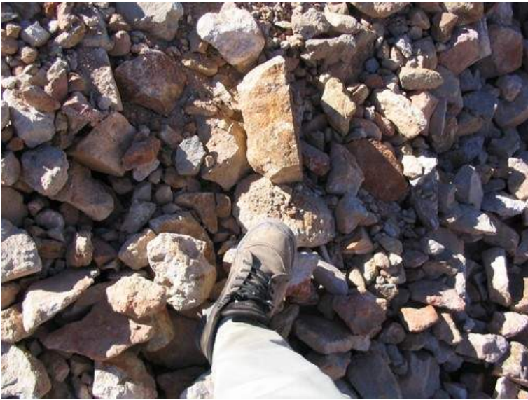
Figure 6. Fill material used for the crusher wing walls
