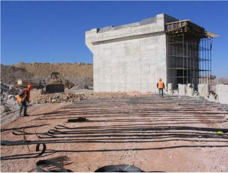
Figure 3. Unwrapping the coils and connecting the strips to the panels
