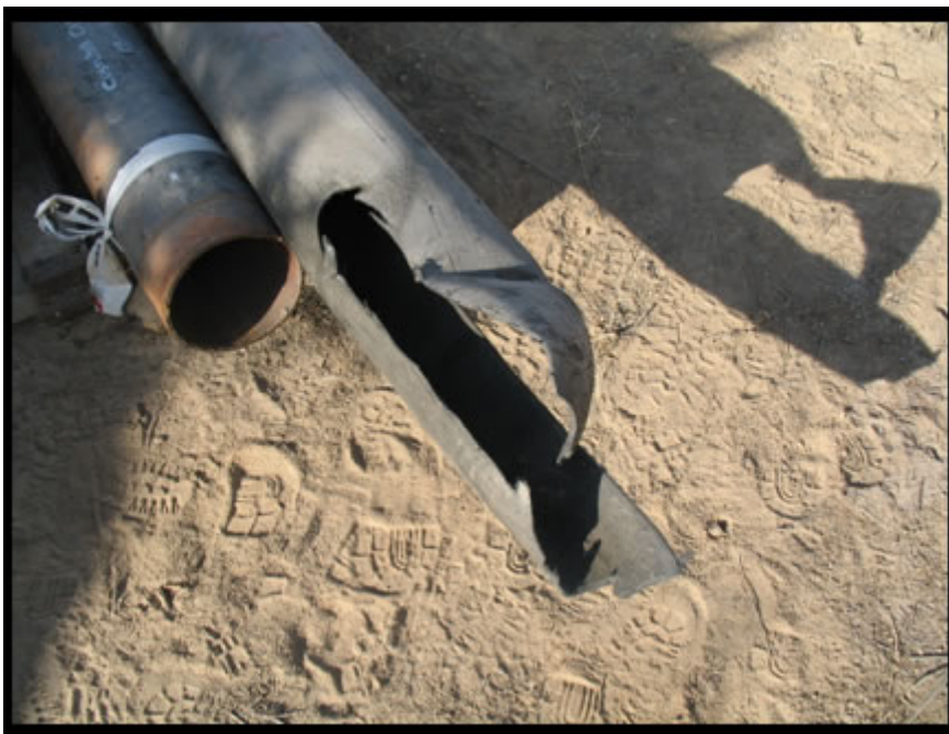
Figure 3. “Beak” fracture in HDPE liner
