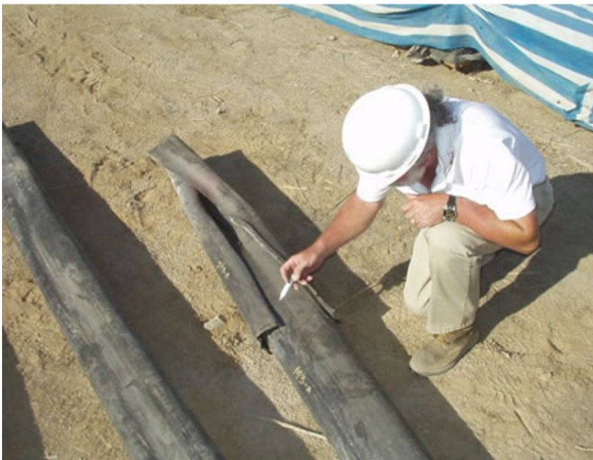
Figure 1. Marking overlapped liner before separating
