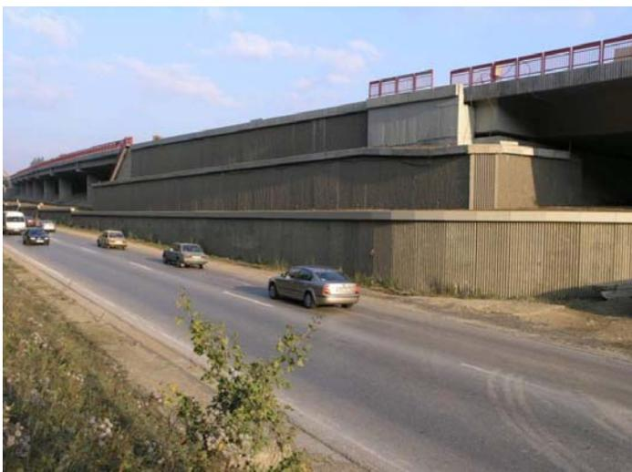
Figure 1. General view of three-tier surface geogrid reinforced wall
