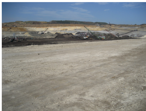
Fig. 7 Excavated slope in the improved soft soil masses, slope inclination 1:6, in the front part uncovered roof of coal layer
