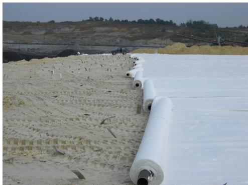
Fig. 5. Installation of geotextile reinforcement on the top of working platform, UTS = 1600 kN/m
