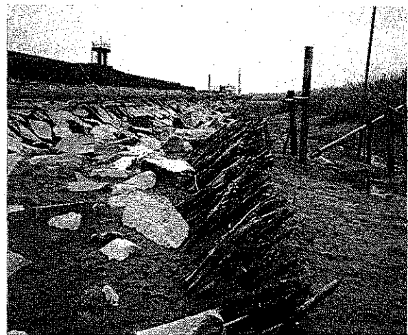
Fig.8 The use of fascines for a sea-side dyke construction, Kyushu, Japan, 1987
