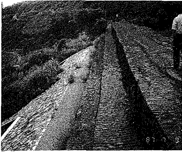
Fig.12 Polymer-grid gabion wall built in 1983, Hong Kong
