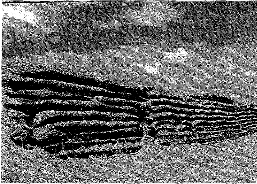
Fig.2 West end of the Great Wall built of soil, reeds, etc. ("The Great Wall", Sunday Mainichi Press Co., Spec. Vol., photographed by A. Yaguchi, 1991, p.120)
