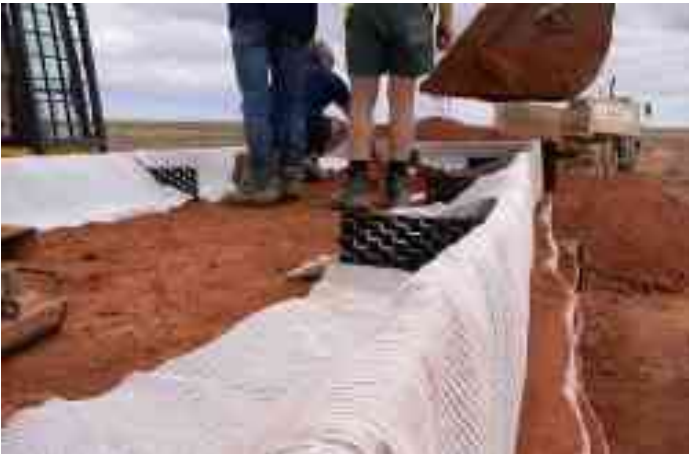
Figure 9: Geotextile Layer Folded Back after Compaction of \frac{1}{2} Layer of Soil
