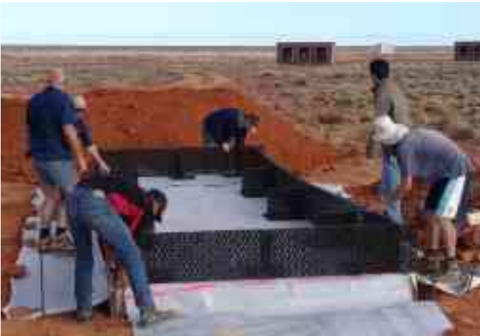
Figure 8: Placing of GeoBlocks on top of Geotextile Layer
