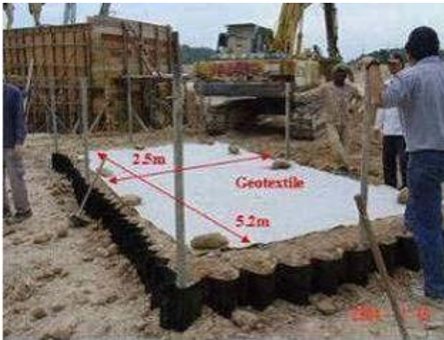
Figure 3: Geotextile Layer for RSW9
