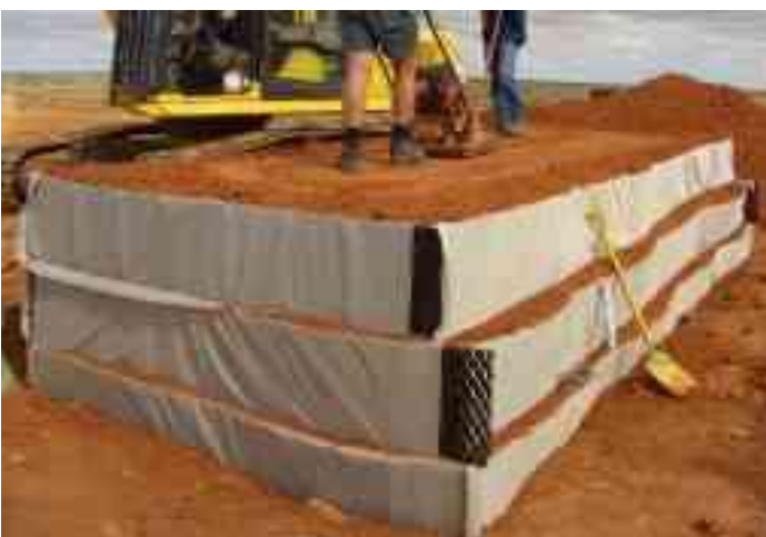
Figure 10: Completed GeoBlock Wall Layer
