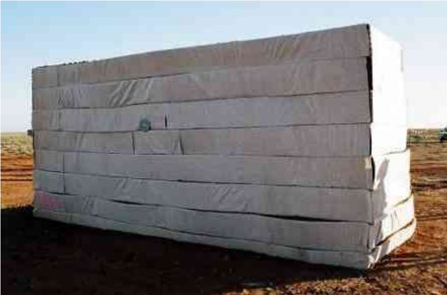
Figure 11: Completed GeoBlock Wall (Front View)
