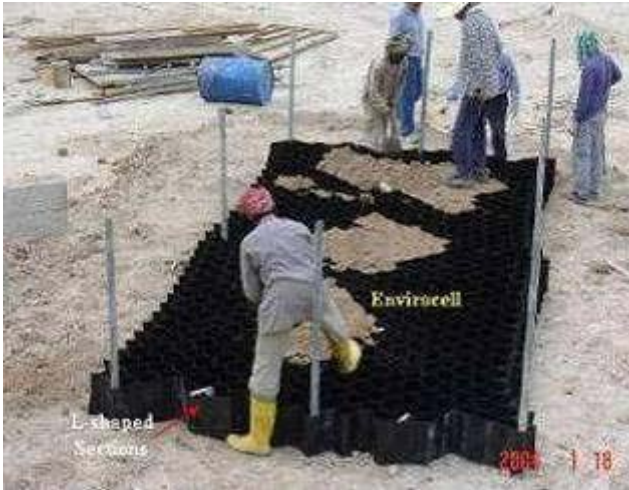
Figure 2: Laying of Envirocell for RSW9
