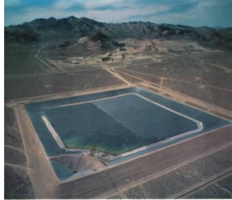
Figure 1 – Geomembrane-lined gold tailings impoundment cell contained by a compacted earth fill tailings starter dam embankment in Nevada, USA in 1988.
