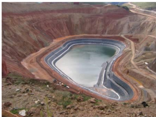
Figure 3 – Geomembrane-lined tailings impoundment for 2004 startup conventional tailings slurry disposal within a depleted open pit gold mine in 2004 in Asturias, Northern Spain.
