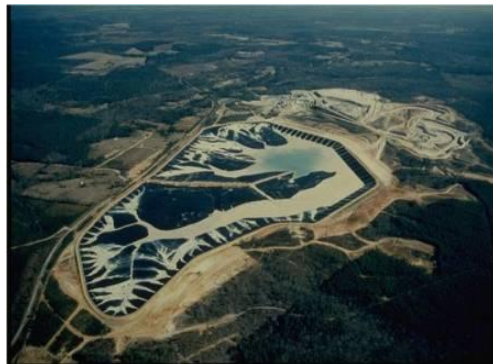
Figure 4- Geomembrane-lined gold tailings impoundment contained by a compacted earth fill tailings dam embankment in South Carolina, USA, in 1987.
