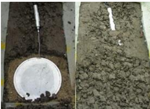
Figure 4. Pressure cell before burying (left) and prior to compaction (right).
