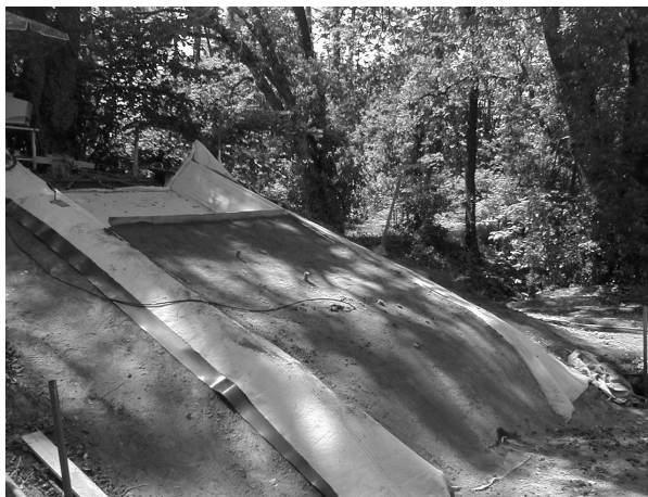
Figure 4. Installation of the protective soil cover in the second experiment.
