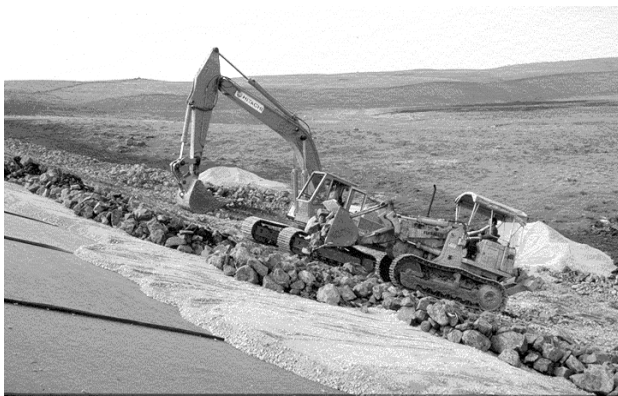
Figure 1. Installation of a geosynthetic system on the face of a dam
