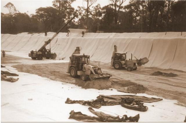
Figure 4. Waratah Road Cell being lined using twin GCL wall and base.
