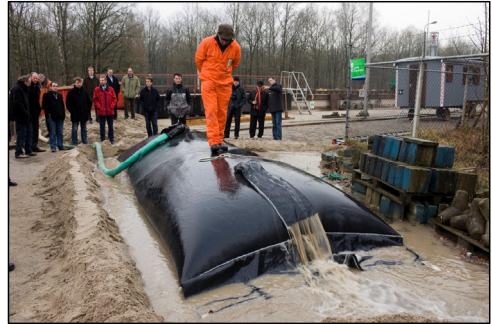
Figure 5. Filling of a geotextile tube (besides the flume)
