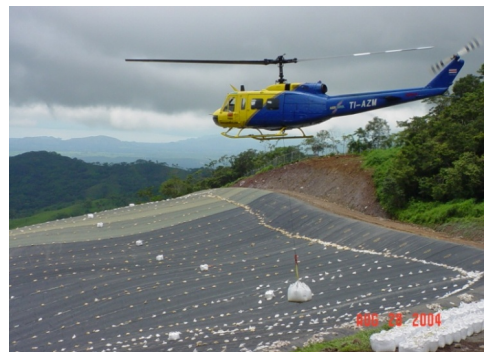
Figure 5: Placement of heavy ballast on installed geomembrane to prevent uplift.
