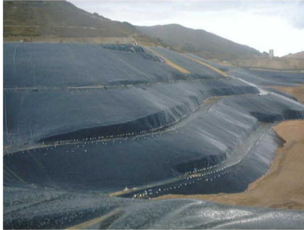
Figure 1: Intermediate benches in steep slopes geomembrane lined leach pad.
