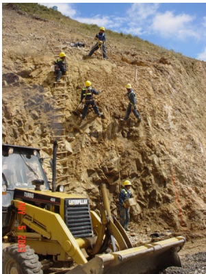
Figure 3: Near vertical cut slope.
