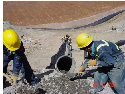
Figure 5: Dual wall HDPE pipe used as a chute.
