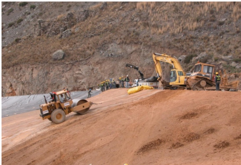
Figure 4: Compaction in a very steep slope.
