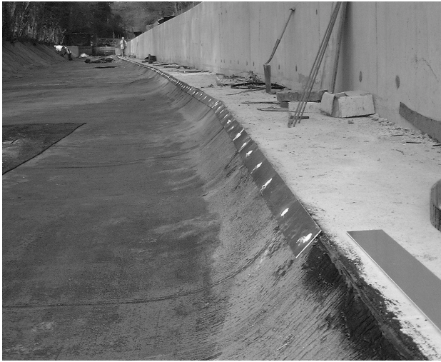
Figure 7: The geomembrane bonded to wall and reinforced
