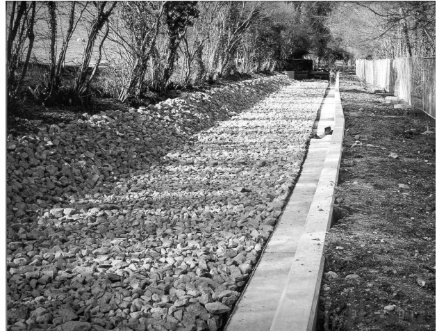
Figure 8: The rip-rap placed along the bed and up the bank
