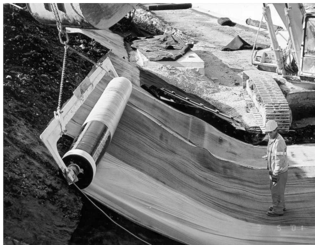
Figure 5: Unrolling the geomembrane
