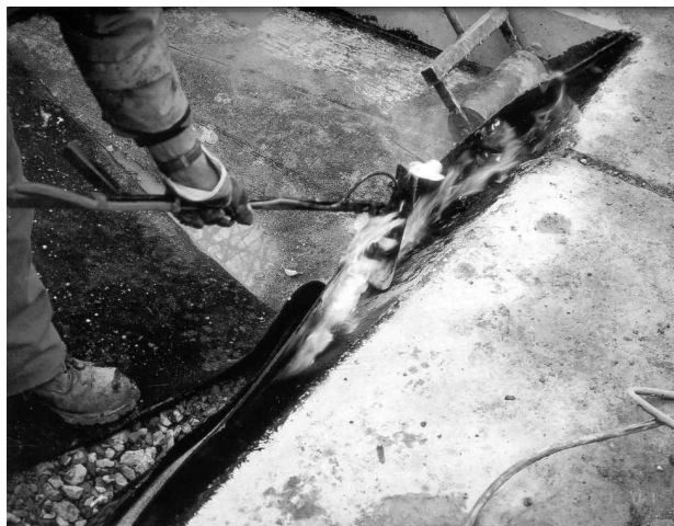
Figure 6: Bonding to the concrete wall
