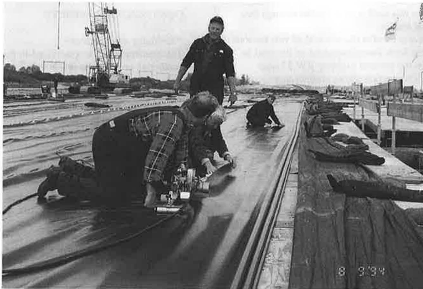
Photo 2: Welding the membrane
