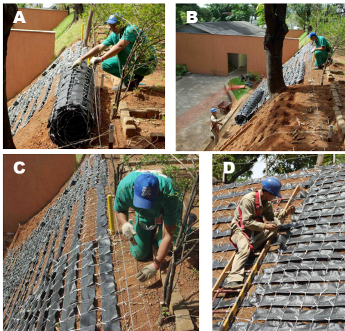
Figure 5 – Procedure to install the netting
