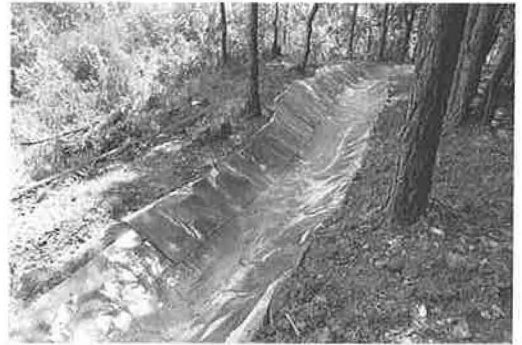
Photo 4: Lining Inaccessible Ditch with Bituminous Geomembrane
