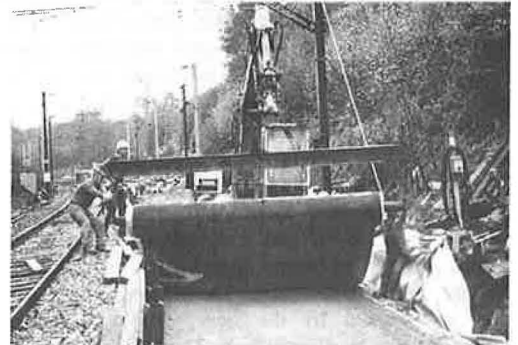
Photo 5: Unwinding Geomembrane from Roll for New Track
