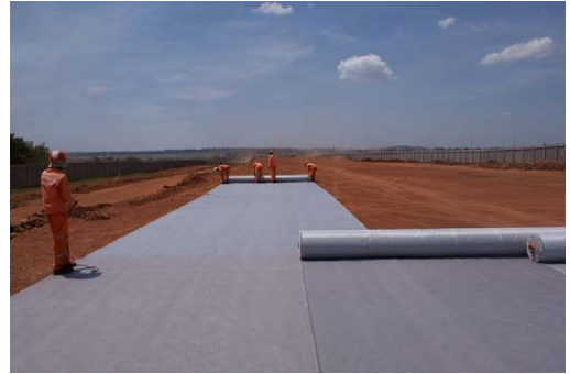
Figure 6: Laying composite geotextile
