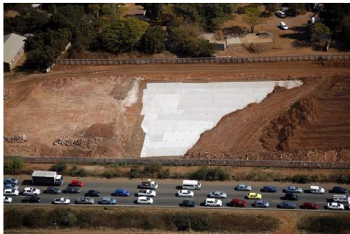
Figure 7: Aerial view of multi-layer geosynthetic-reinforced embankment during construction
