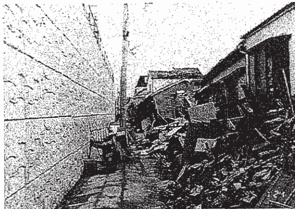
Fig. 25 View in front of the GRS-RW immediately after the earthquake
