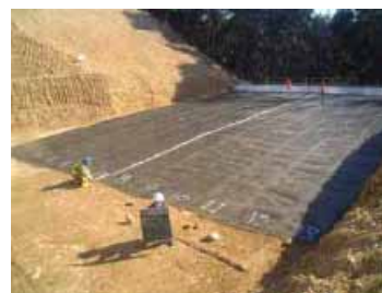
Fig.7. Installation of geogrid layers
