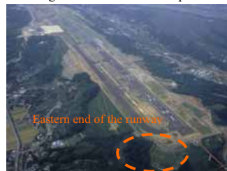
Fig. 2. A view of the completed airport and locations of the GRS-RWs
