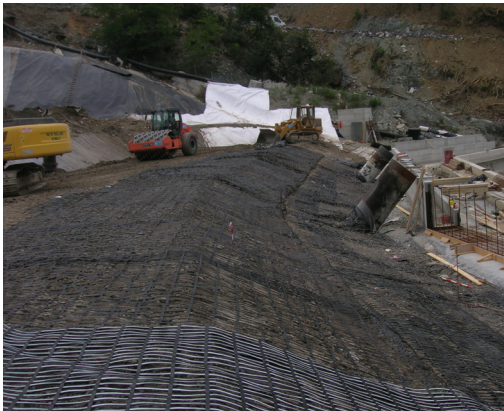
Figure 1 Construction stage of the embankment.
