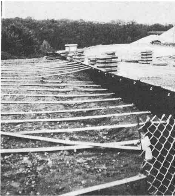
PHOTO 4 REINFORCED EARTH STRIPS, TEST WALL NO. 1
