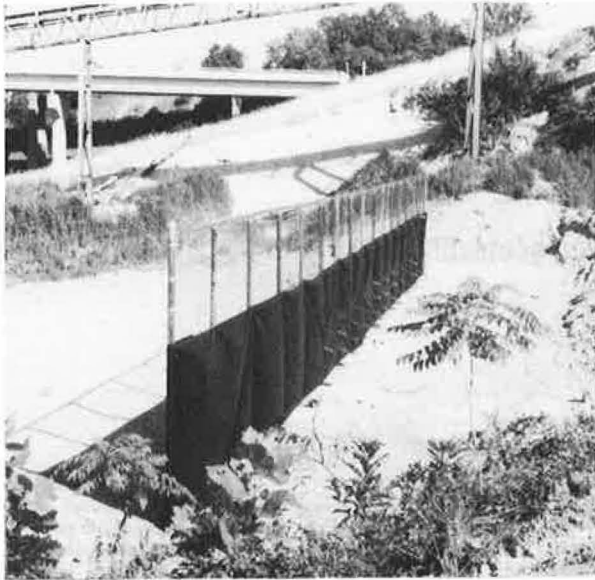
PHOTO 2 TEST WALL NO. 3, BEFORE BACKFILLING
