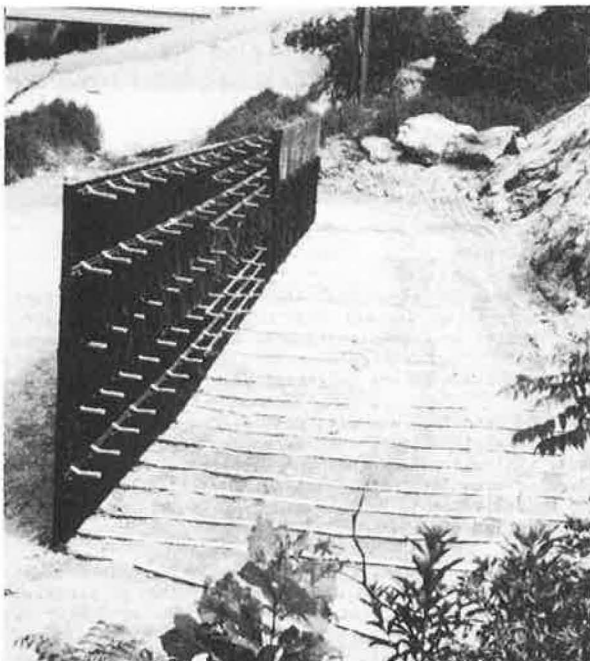
PHOTO 7 READY TO START BACKFILLING, TEST WALL NO. 3
