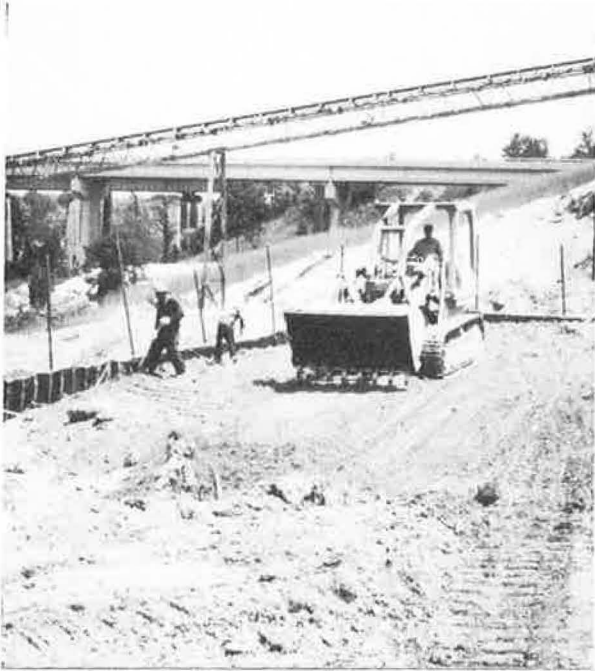
PHOTO 10 COMPACTING BACKFILL, TEST WALL NO. 2
