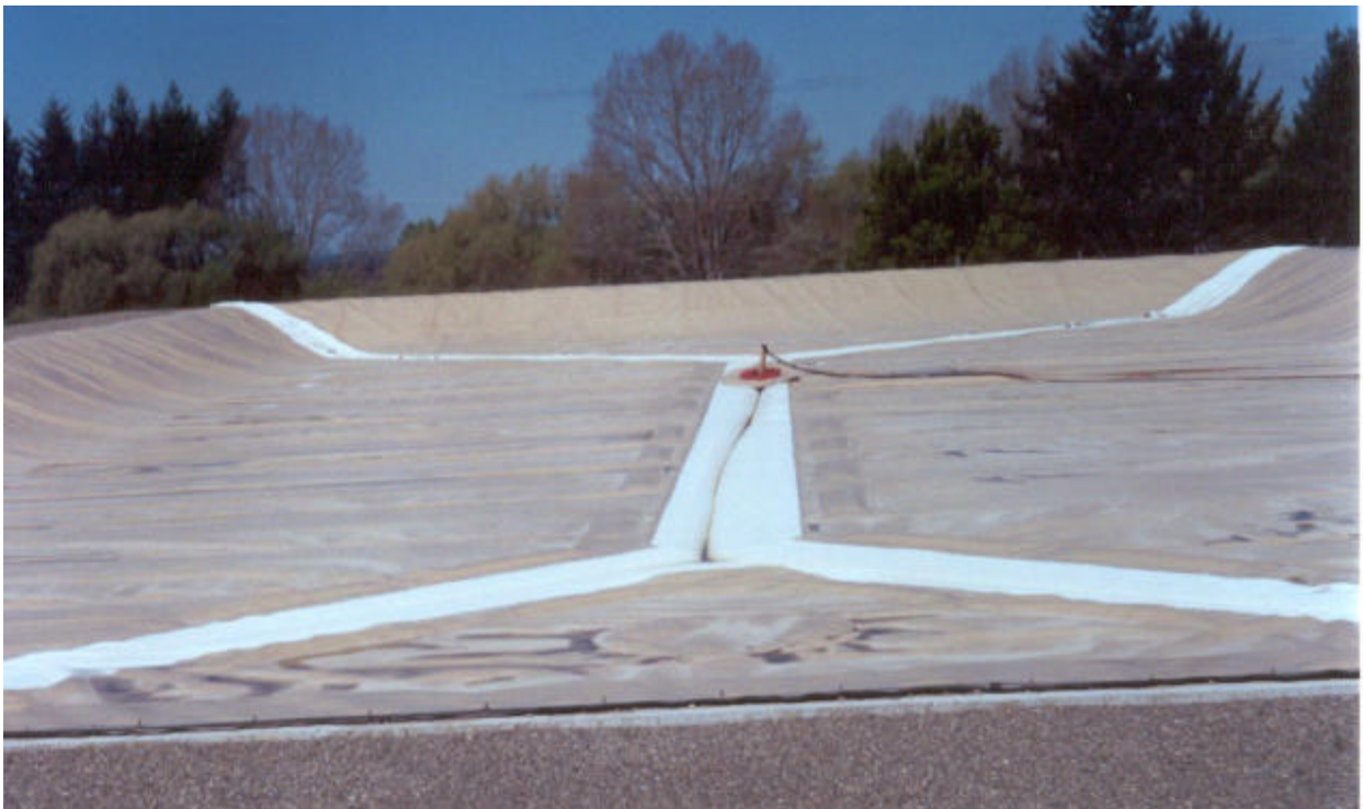
Figure 5. Waimate Reservoir on completion
