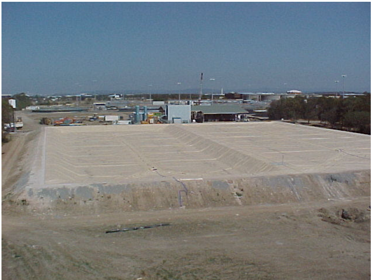
Figure 3. Completed Luggage Point Covers. Note hinges same colour as main plate.
