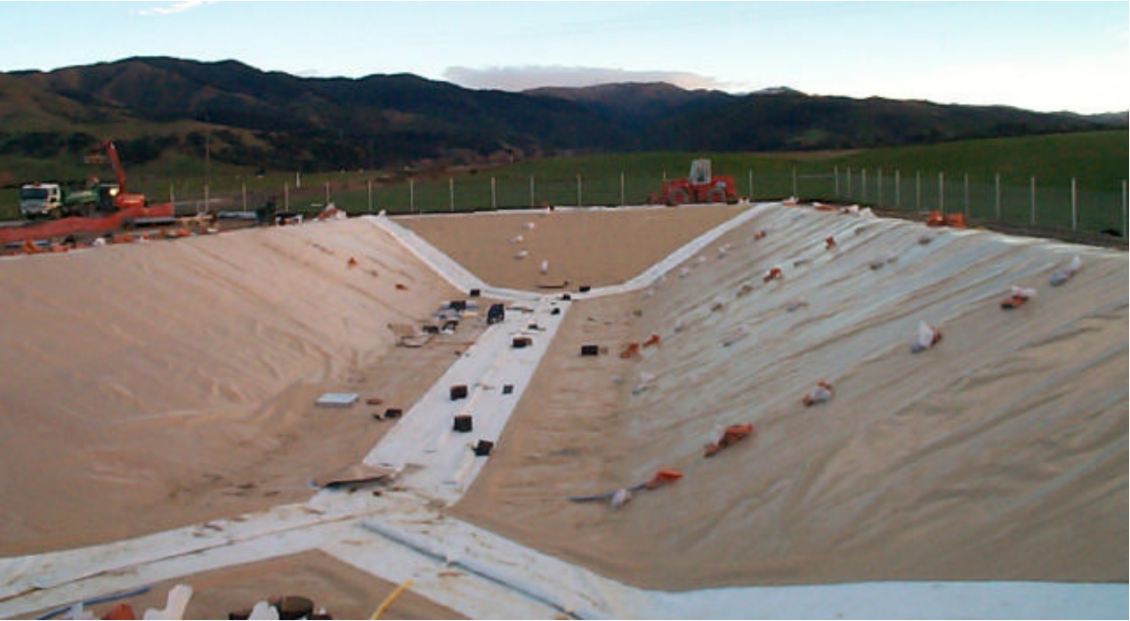
Figure 4. Waimate Reservoir during construction
