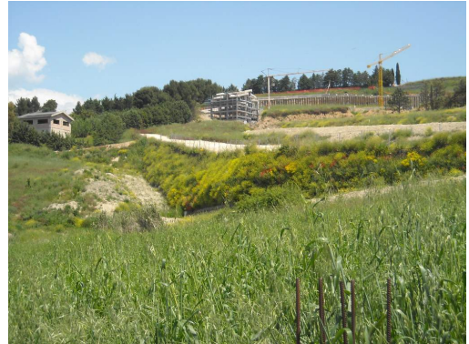
Photo 4. Buildings construction beginning
