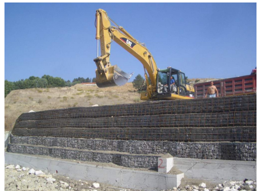
Photo 2. Phase of reinforced steep slope carrying out
