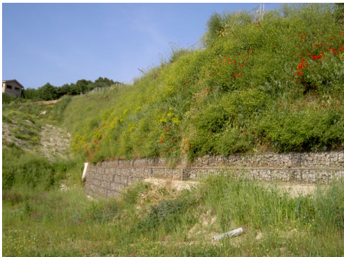
Photo 3. Vegetation revival on reinforced steep slope frontage 1 year later
