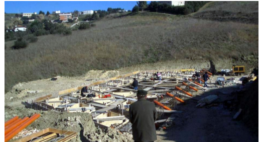
Photo 1. Foundations basement construction
