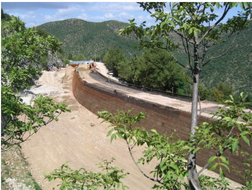
Figure 7. Trapezoidal embankment during construction (basin side inclined 80°)
