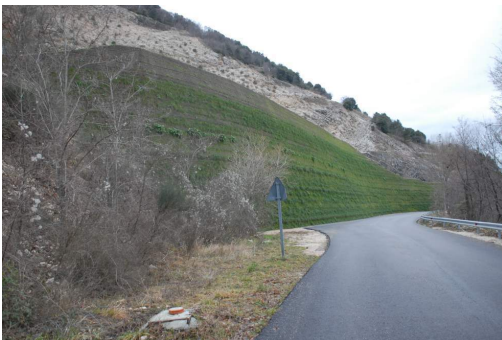
Figure 8. Final situation at the road side (front slope 65°)
