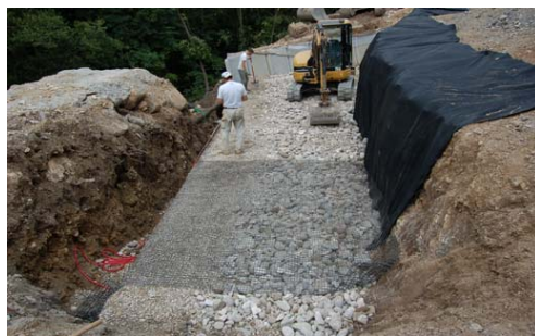
Figure 3. Bottom foundation layer filled with rounded cobblestone wrapped with woven filter.
