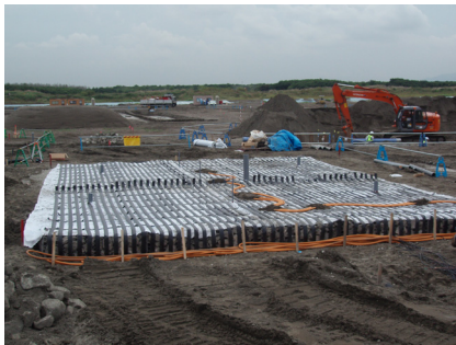
Figure 2. Mattress construction
