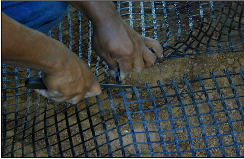
Figure 08 – Geogrid installation
