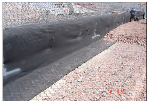
Figure 07 – Geotextile installation
