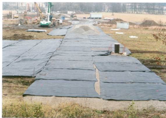
Figure 2. Dobrany. Geotextile-reinforced embankment base
