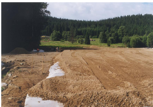
Figure 1. Strazny. Embankment base reinforced with geotextile
