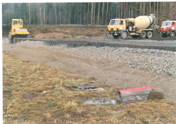
Figure 6. Dobrany. Finished road on peat
