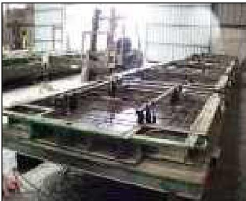
Figure 3. Loops in place before casting
