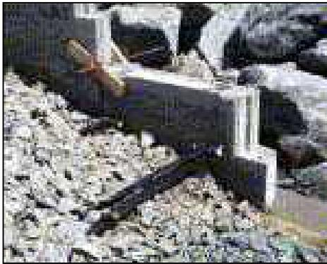
Figure 2. A PARAWEB V strip connected to the synthetic connection
