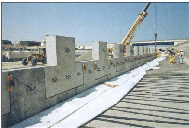
Figure 7. MAJAS canal during construction
