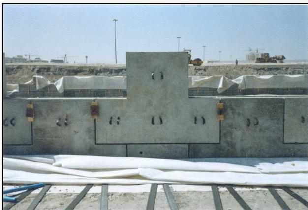
Figure 8. Rear view of panels with attachments
