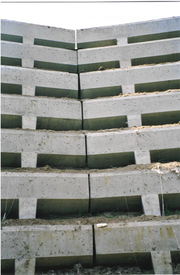
Figure 5 - Close up of Corner Detail - A view of the inside corner from below to demonstrate the exact fabrication and erection of the wall even in this three dimensional environment of rough earthworks.
