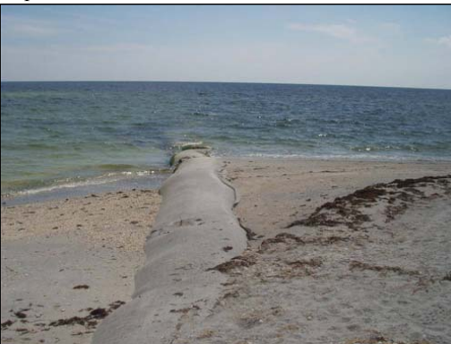
Figure 3. Low profile geotextile tube groin, Stump Pass, Florida.
