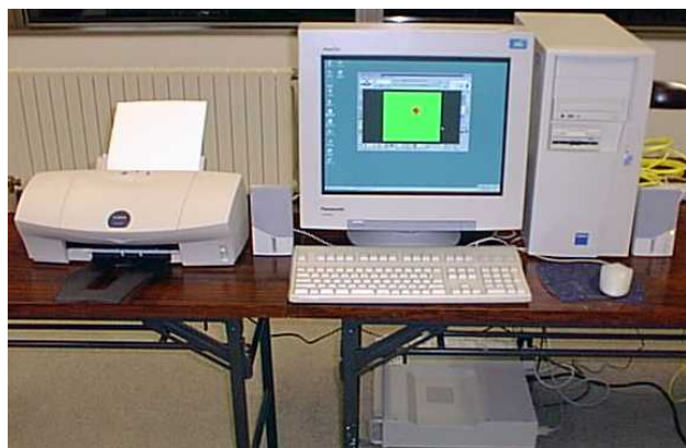
Photo 3. Permanent ELL system at on-line configuration. Desktop PC computer at control room 24 hours drives the 11 measuring units situated outside and located at perimeter of landfill. The failure is immediately detected and its position is precisely computed and displayed on the screen. The alarm is appeared at the same time.
