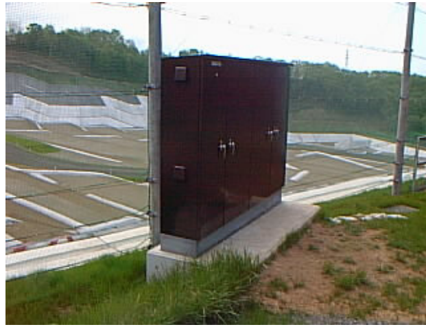
Photo 1. Permanent ELL system at on-line configuration. (Otaru municipal landfill, Japan – 80,000 m 2 ). 4 central boxes comprising of 11 measuring units are situated outside and located at perimeter of landfill. The communication between these units and PC desktop computer
