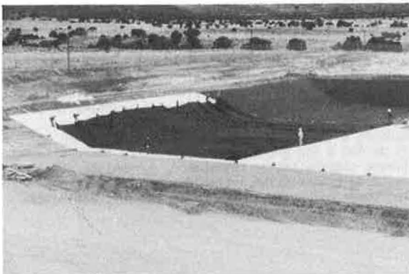
Figure 1. Photograph of Butyl Geomembrane Being Installed Over Polypropylene Geotextile.
