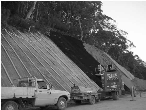
Figure 11 Flat drainage installed the full slope length followed by cellular confinement.
