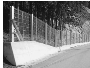
Photograph 2. An existing stone guard fence
