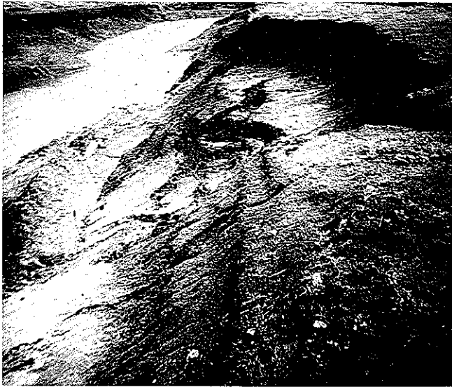
Figure 4 R.H.S. Slip at 37.50 Km
