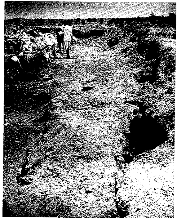
Figure 8 Major Slip Bank Details at 36.90 km.
