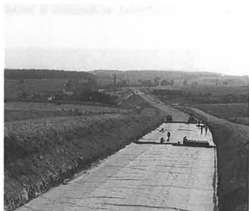
Photograph 2. Installation of the lining system on the Vittel bypass.
