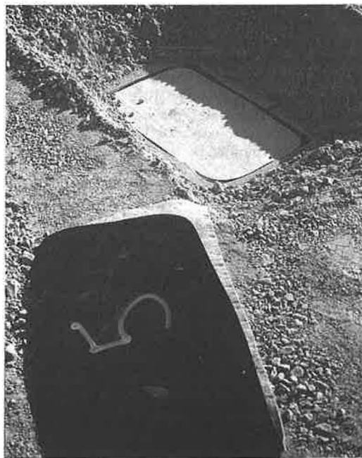
Photograph 1. Sampling of geomembrane on the pilot test. Vittel bypass.
