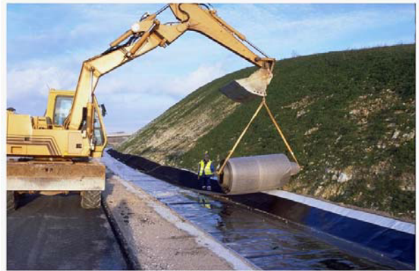
Figure 5. Installation of the three-dimensional geotextile
