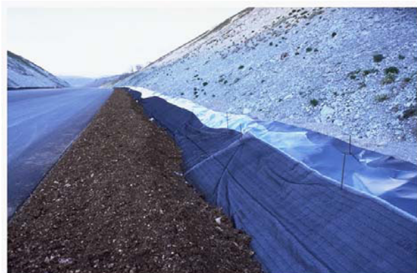
Figure 3. installation of soil protection
