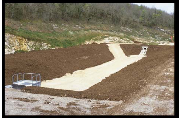
Figure 4. Basin with its soil protection
