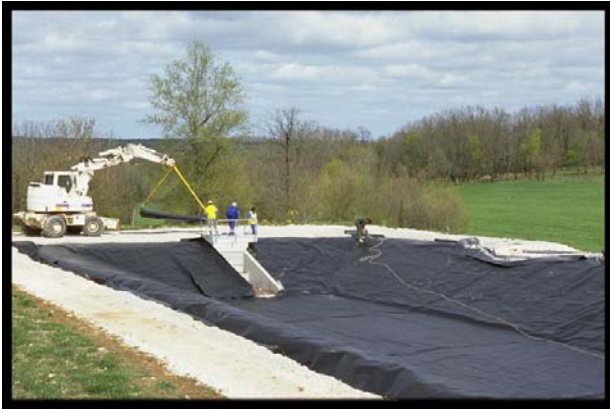
Figure 1. Installation of HDPE geomembrane on a basin.
