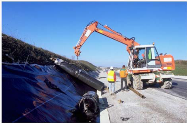
Figure 2. Installation of elastomeric bituminous geomembrane in the channels
