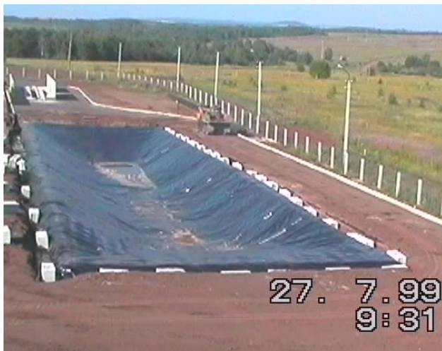
Fig. 2 The isolated trench before filling
