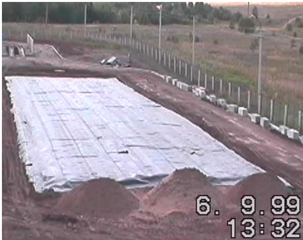
Fig. 3 HDPE envelope around polluted soil
